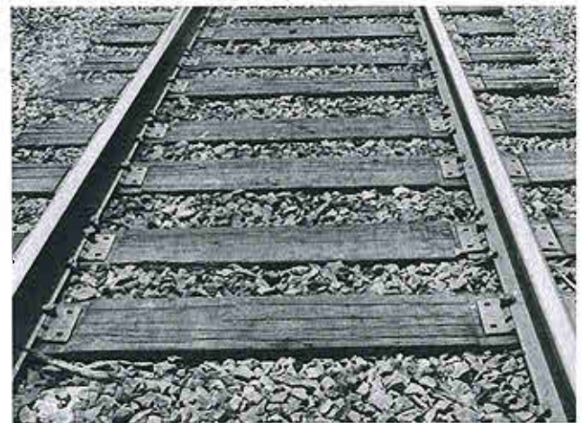
7" x 12"—8' 6" two-piece, dowel-laminated ties.
