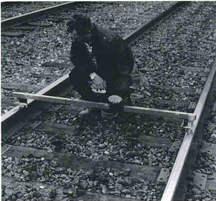
Measuring gage and cross-level.
