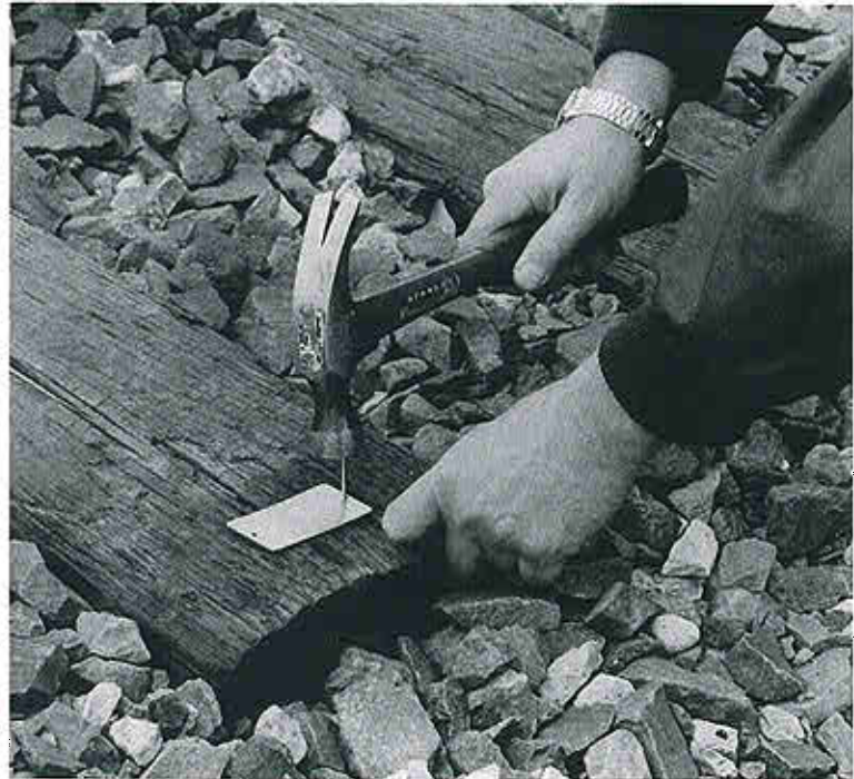
Tagging for tie identification.
